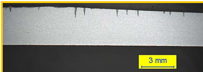
Fig.7: Cross section 1 (cut out from ground and polished area). Several wedge-like cracks, starting from outside/gas-side, could be observed. The cracks were filled with oxides/corrosion products. Etched with nital.
